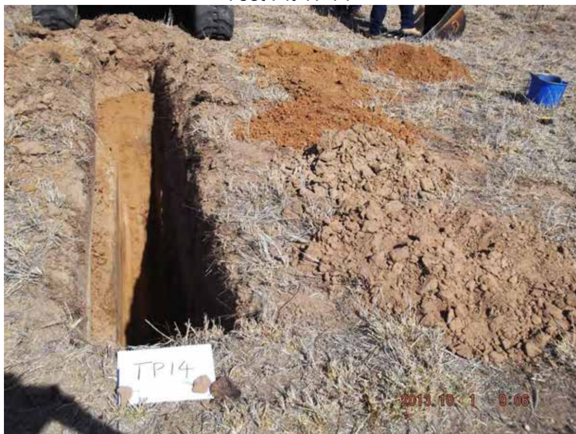
Test Pit TP14
