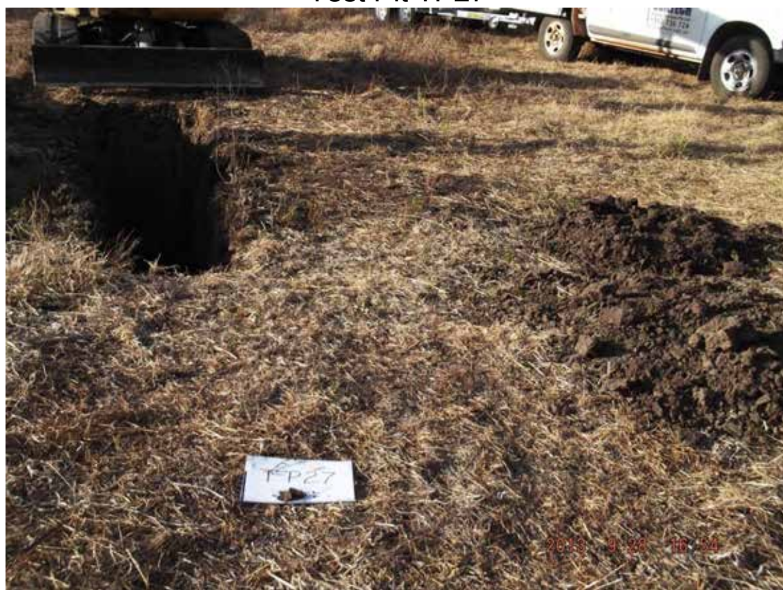
Test Pit TP27
