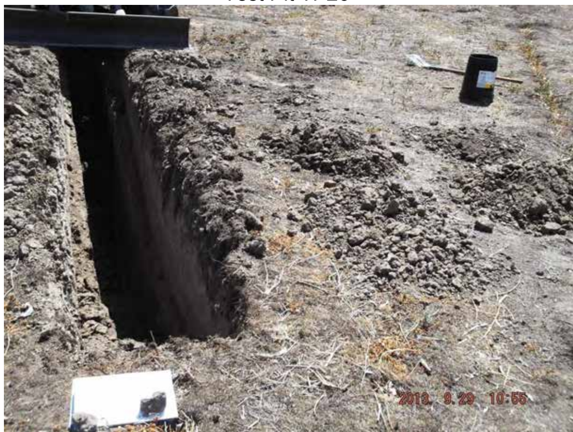
Test Pit TP26
