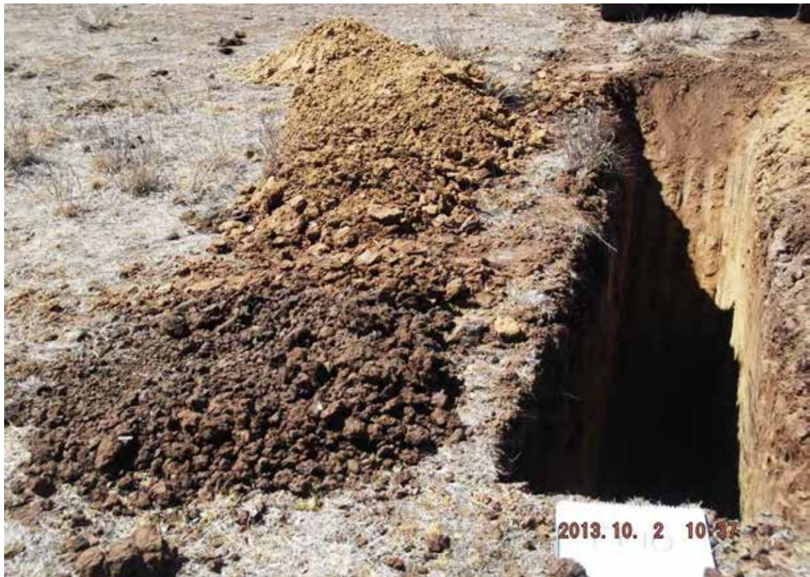
Test Pit TP9
