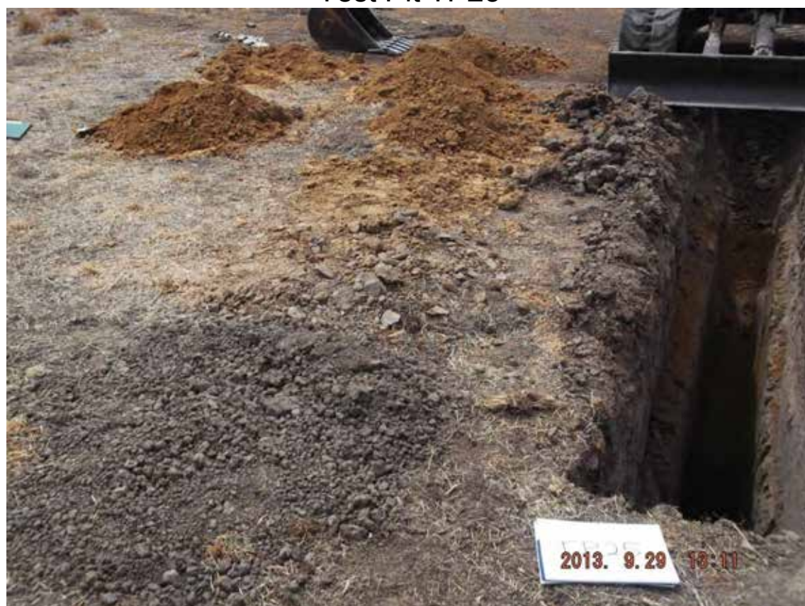
Test Pit TP25
