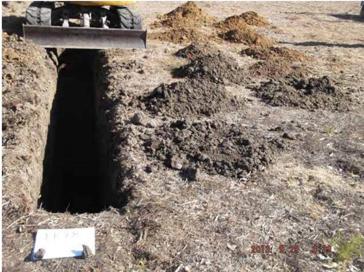
Test Pit TP28
