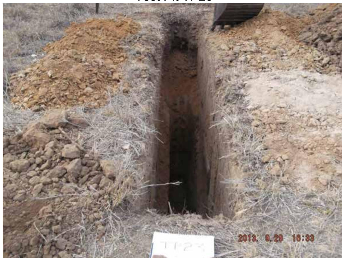
Test Pit TP23
