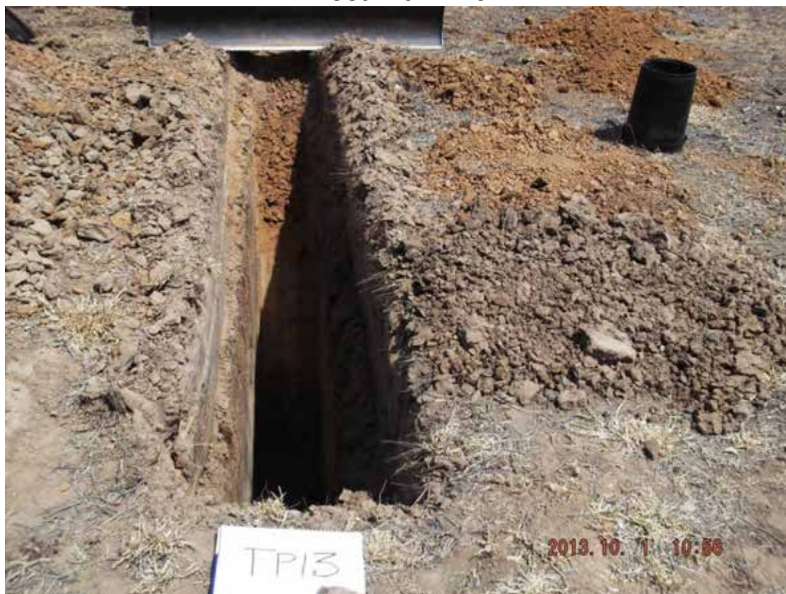
Test Pit TP13
