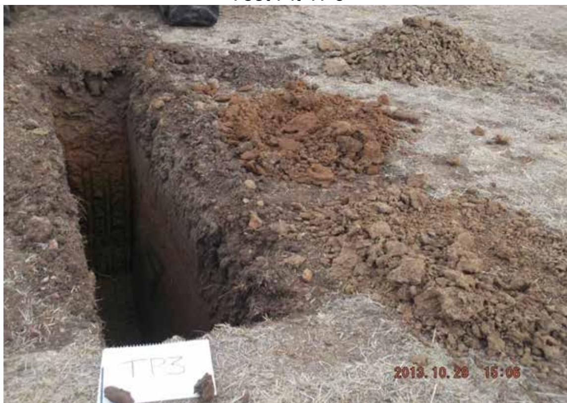
Test Pit TP3
