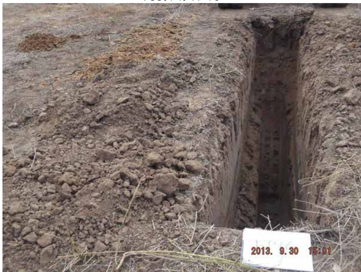
Test Pit TP16
