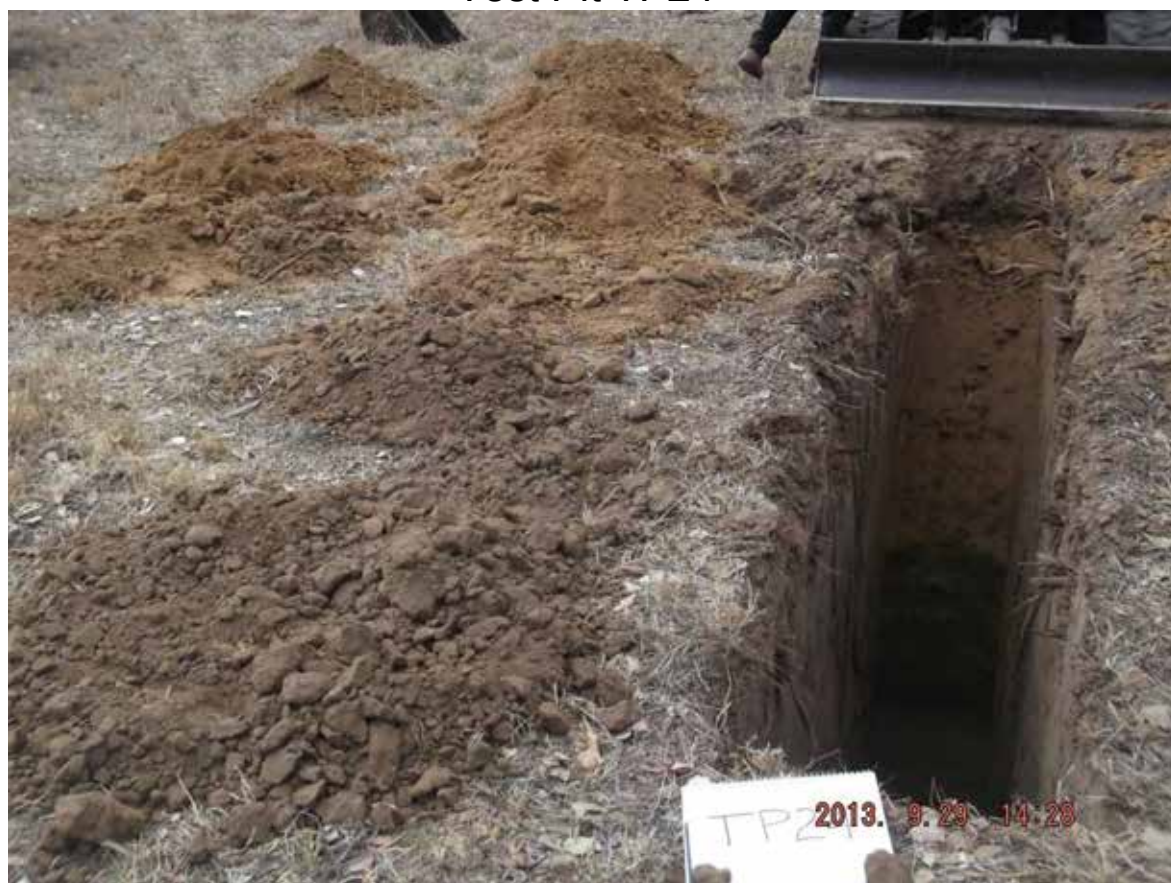
Test Pit TP24
