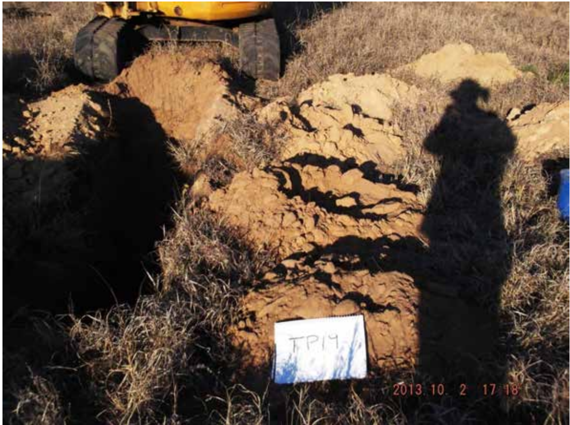
Test Pit TP19
