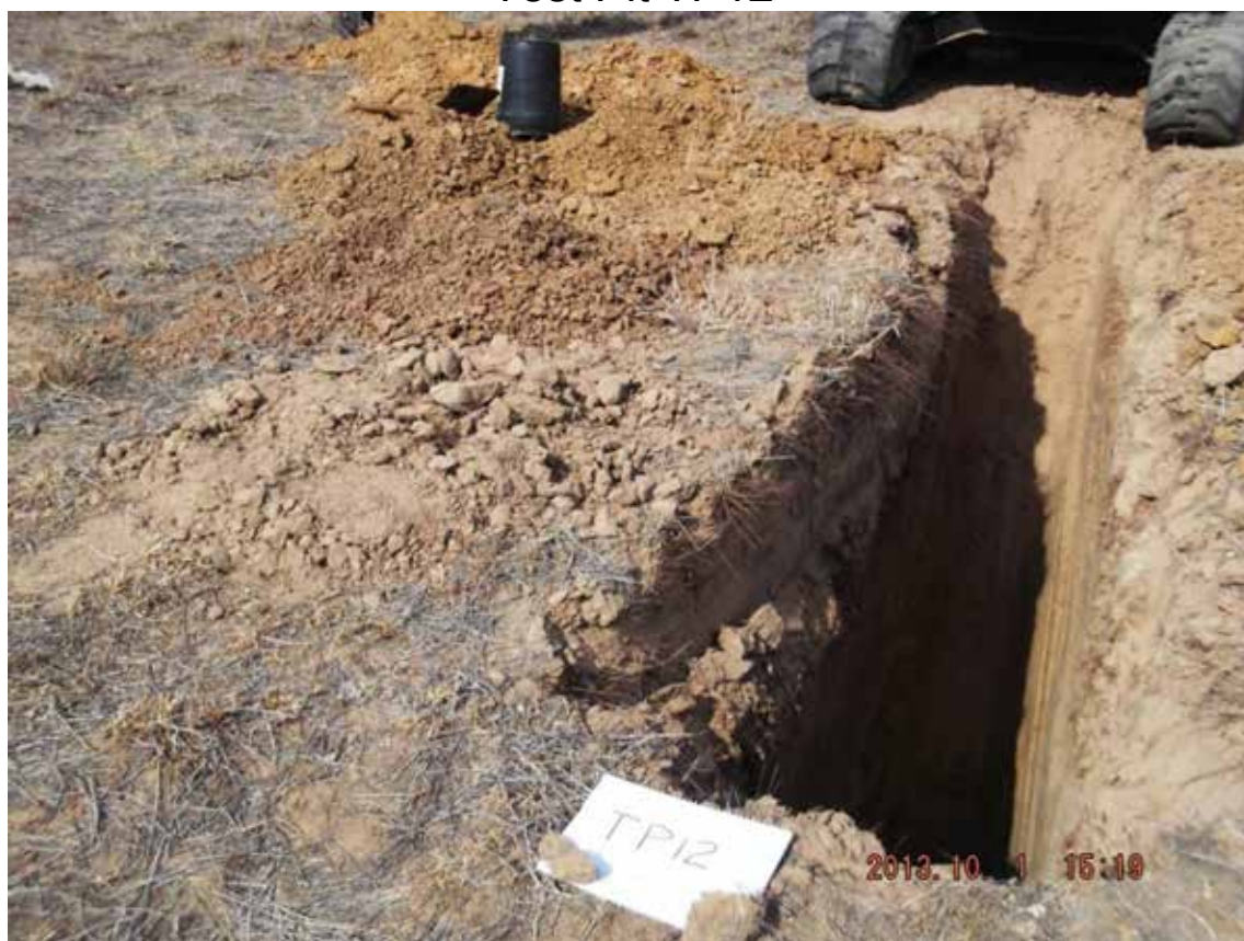
Test Pit TP12
