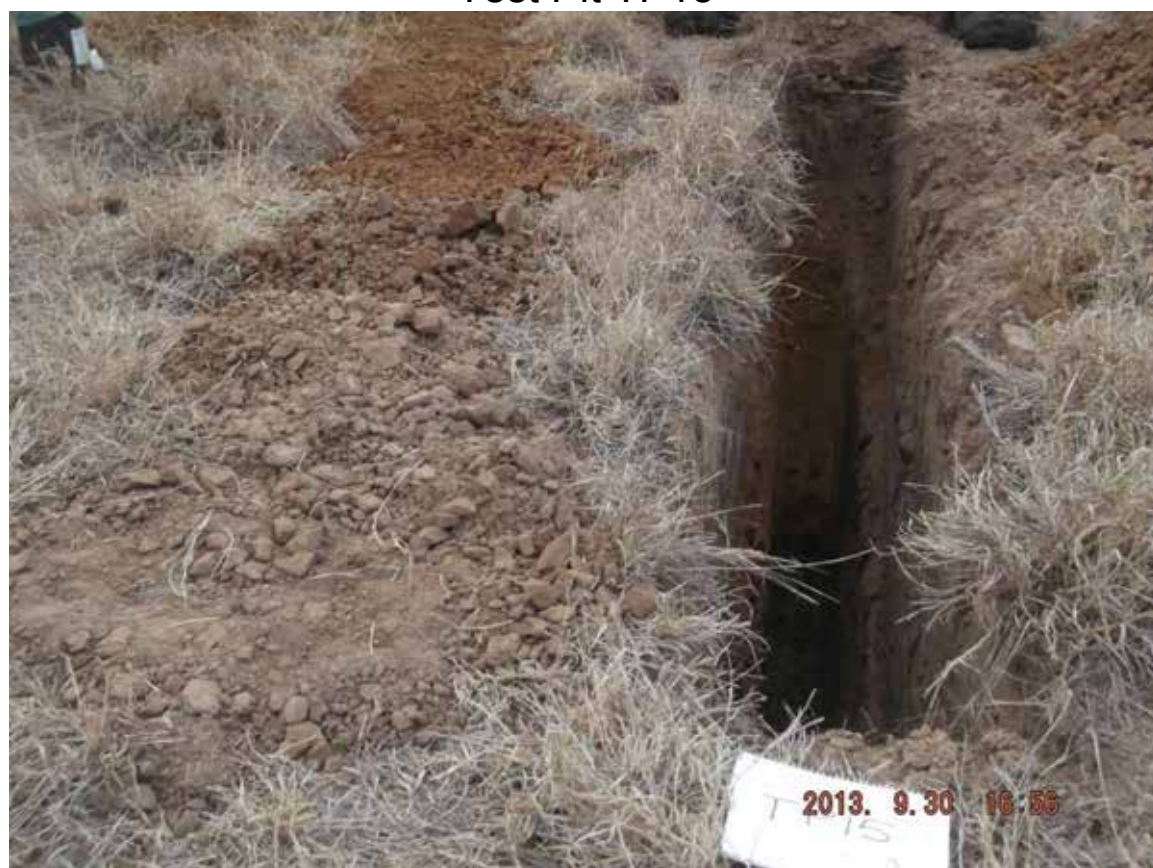
Test Pit TP15
