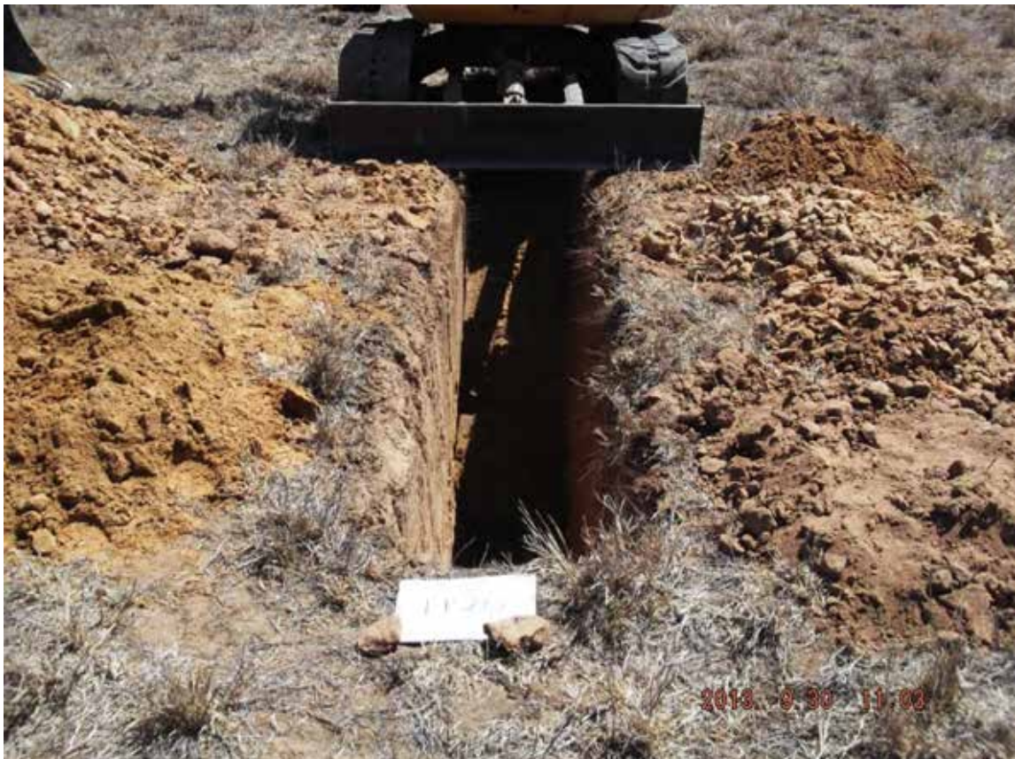
Test Pit TP20
