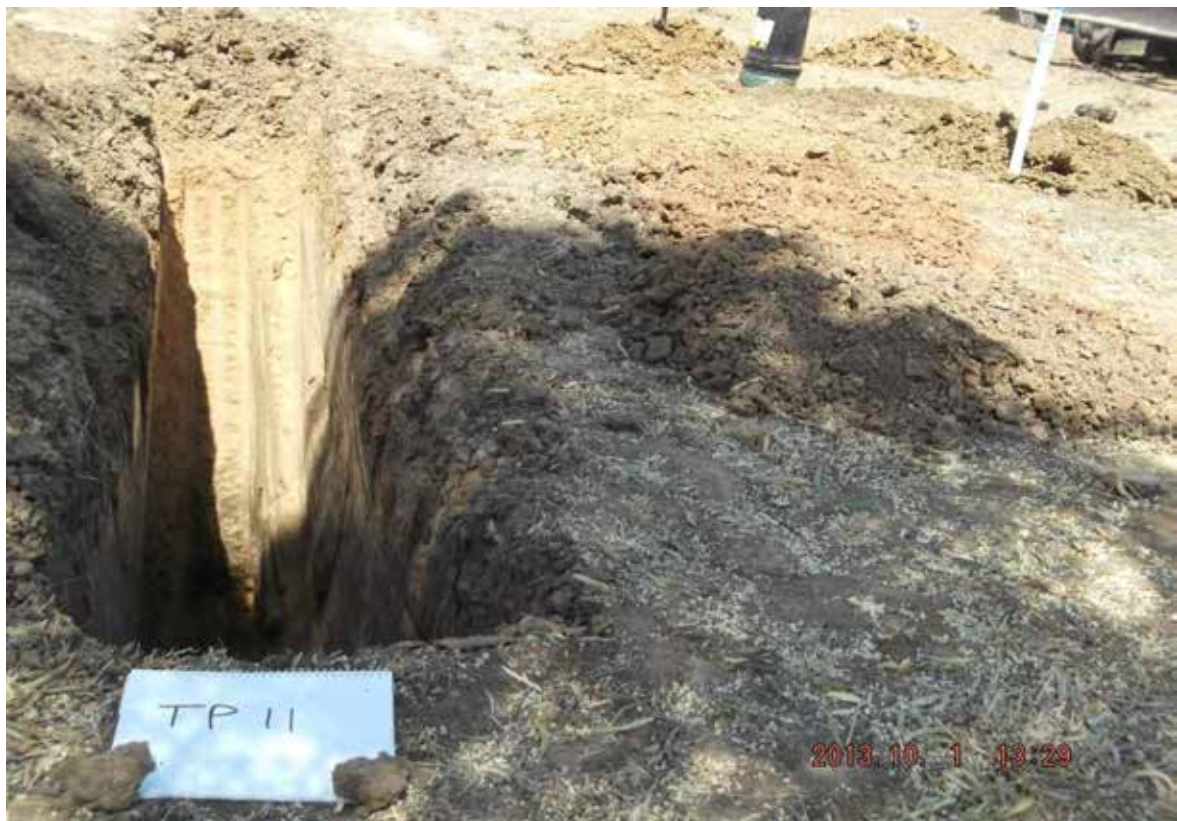
Test Pit TP11
