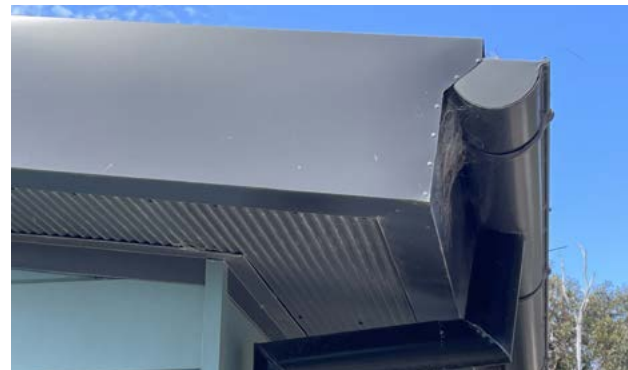
Non-combustible eaves, including soffits (eave lining)
