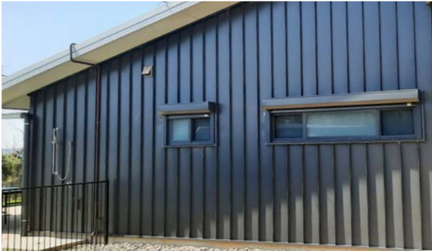
Non-combustible cladding example
