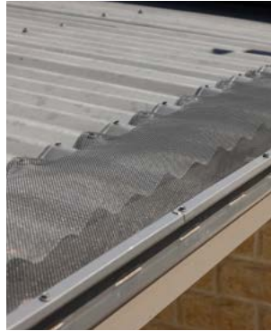
Bushfire rated steel gutter guard with holes less than 2mm
