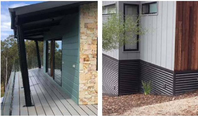
Non-combustible cladding examples
