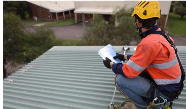
Roof inspection &amp; repairs
