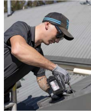
Professional installation of gutter guard
