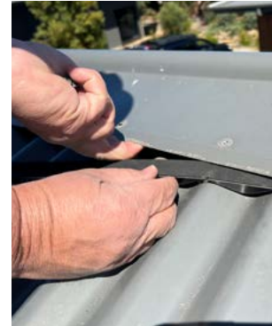
Profile cut ridge insert installation
