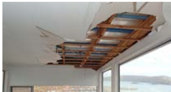
Examples of cyclone damage to Queensland homes
