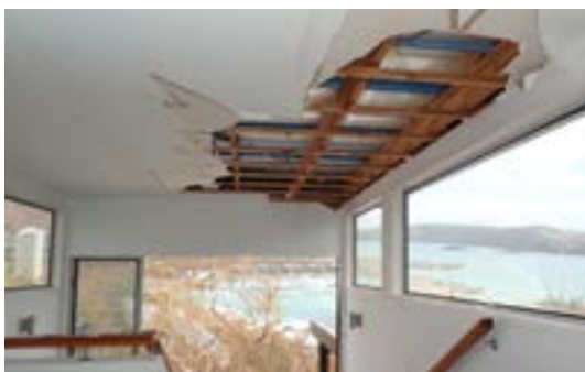
Damage to plasterboard ceiling
