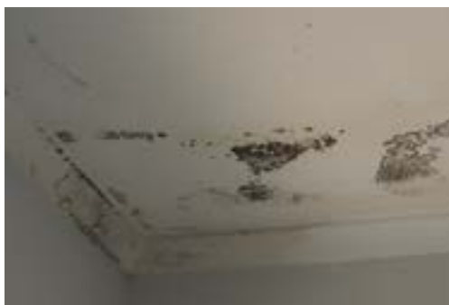
Mould on ceiling
