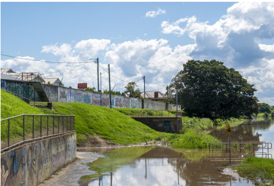
Figure 9. Part of the South Grafton levee system (source: T Weber)
